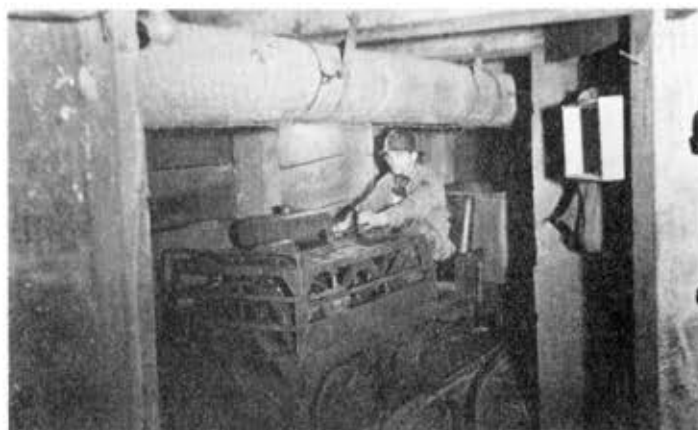
A member of the bridge building gang #22 driving the little ore car that Charles thought was going to be such a keen job.
